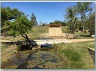
OEI provided the downstream assessment and roadway drainage design for the Pioneer Drive extension, the improvements of which will drain into Wildbriar Lake, which is formed by an earthen dam and has an approximate drainage area of 100 acres. The drainage area is in a rapidly developing area, so OEI assessed the effects the roadway improvements (hydrologic assessment) as well as other development in the area would have on the lake and its ability to convey large flood events.
