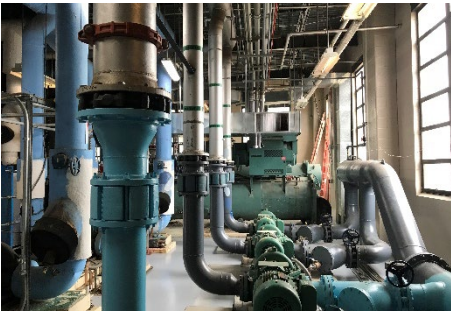
Bonham VAMC Chiller Replacement
