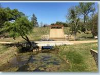
OEI provided the downstream assessment and roadway drainage design for the Pioneer Drive extension, the improvements of which will drain into Wildbriar Lake, which is formed by an earthen dam and has an approximate drainage area of 100 acres. The drainage area is in a rapidly developing area, so OEI assessed the effects the roadway improvements (hydrologic assessment) as well as other development
