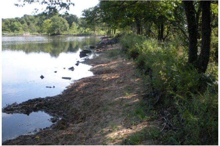
Figure 3 – Neff Lake Dam, Texas, Aug 25, 2010
