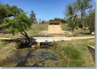
OEI provided the downstream assessment and roadway drainage design for the Pioneer Drive extension, the improvements of which will drain into Wildbriar Lake, which is formed by an earthen dam and has an approximate drainage area of 100 acres. The drainage area is in a rapidly developing area, so OEI assessed the effects the roadway improvements (hydrologic assessment) as well as other development in the area would have on the lake and its ability to convey large flood events.
